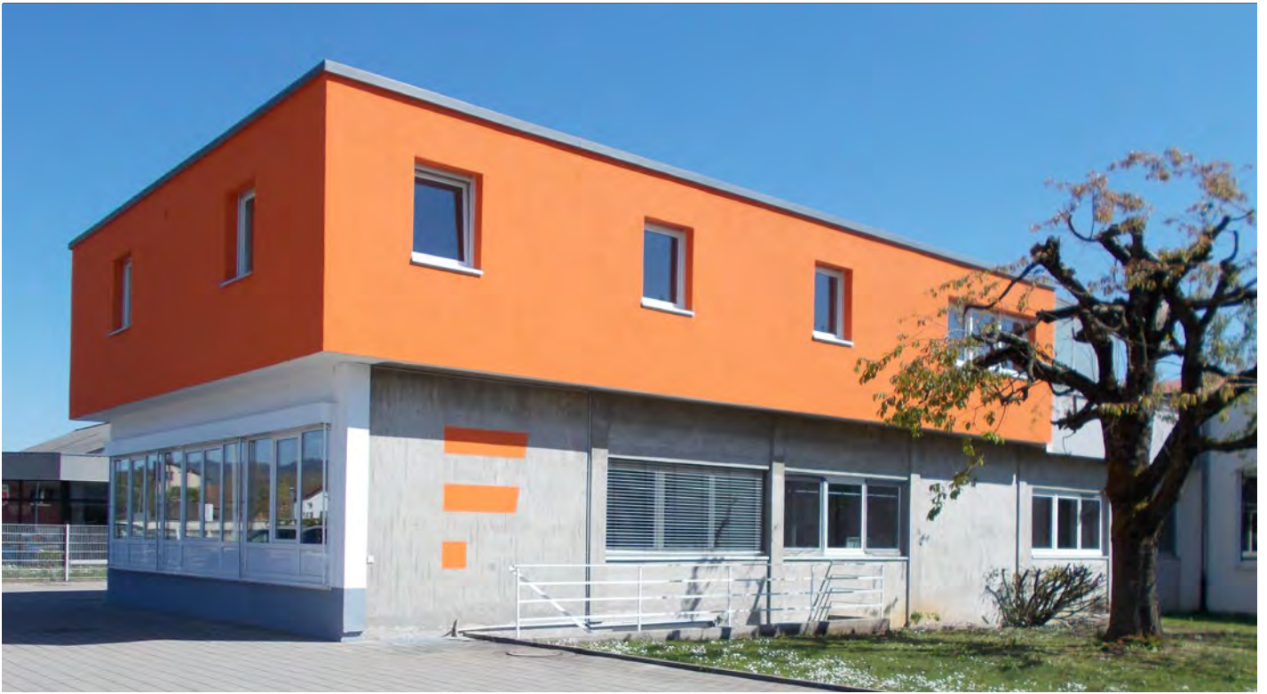
Eye-catcher in Schopfheim. The new value proposition of the Business Unit Labels also includes simply looking great. The freshly painted façade catches the eye.
