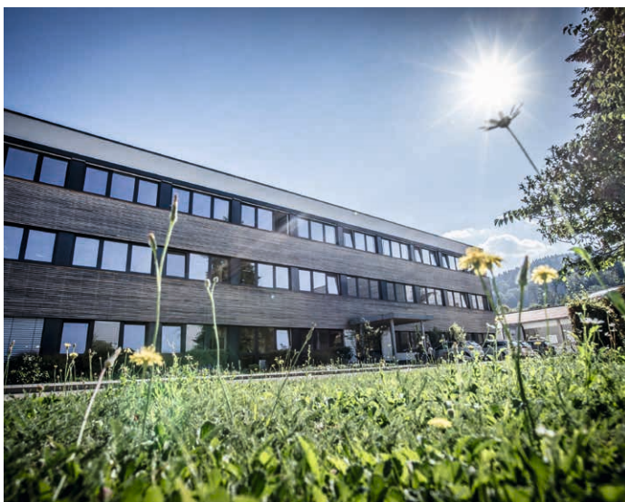
The modular administration building at the company headquarters in Waldkirch can be easily dismantled and integrated into the new building for the move to the Inried industrial park.
