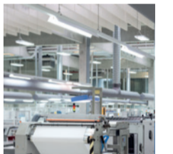
The zone concept with LED lights also saves energy at the Binzen site.
