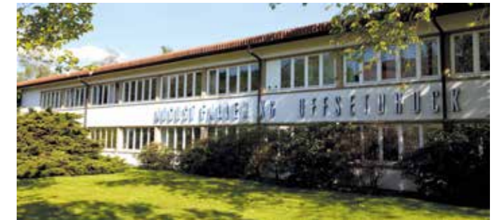
The former administration building in Waldkirch was modernised in 2014
