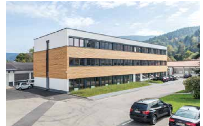
The „system building“ in Waldkirch
